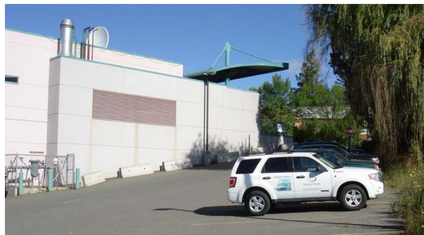
Existing Parking East Lot
