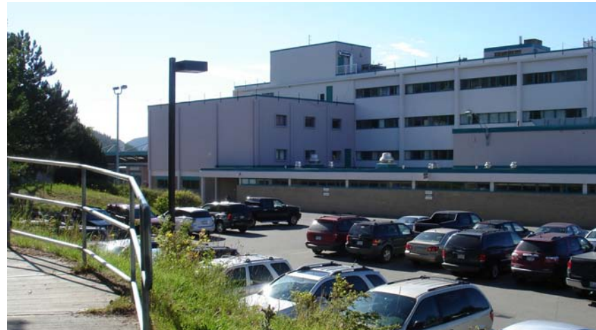
Existing Parking Front
