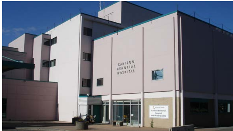
Main Building North Side
