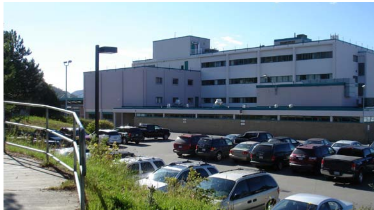
Main Building North Side Inpatient Floors
