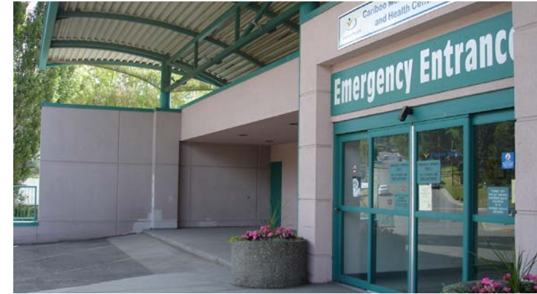
Ambulance Bay and Emergency Entrance
