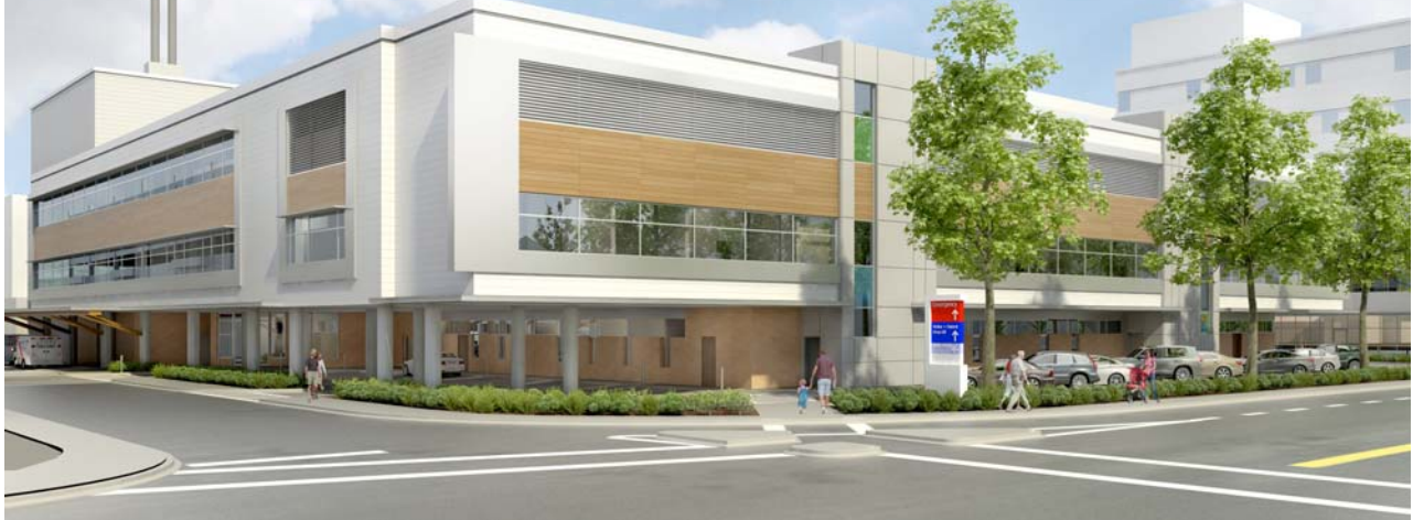
View of the new IHSC Project as seen from Rose Avenue and Pandosy Street
