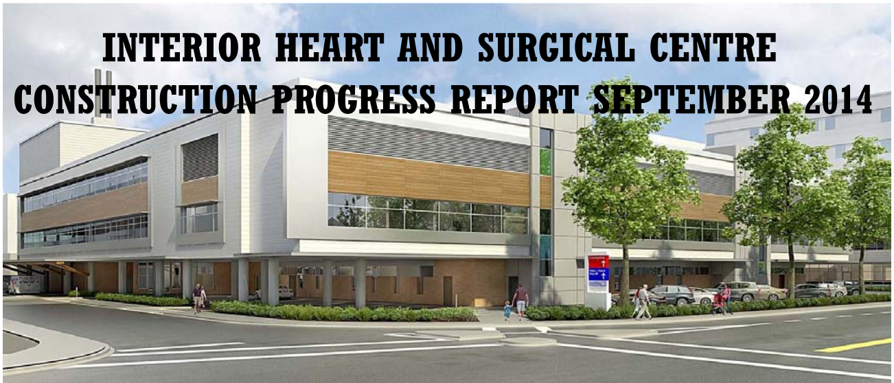
View of the new IHSC Project as seen from Rose Avenue and Pandosy Street
