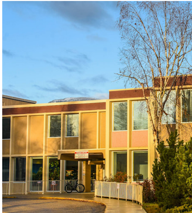
Queen Victoria Hospital in Revelstoke ( Revelstoke Review, 2020 )
