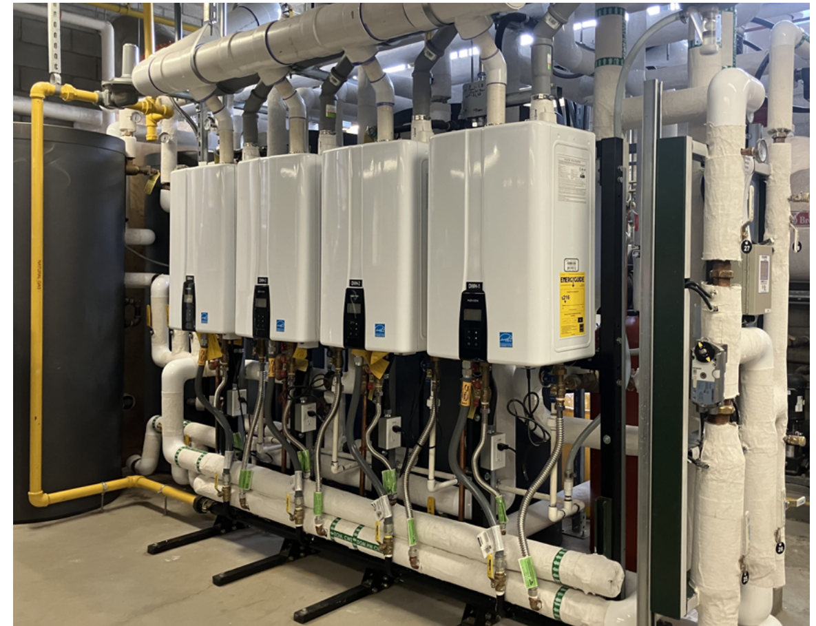
High-efficient condensing domestic hot water heaters at Creston Valley Hospital
