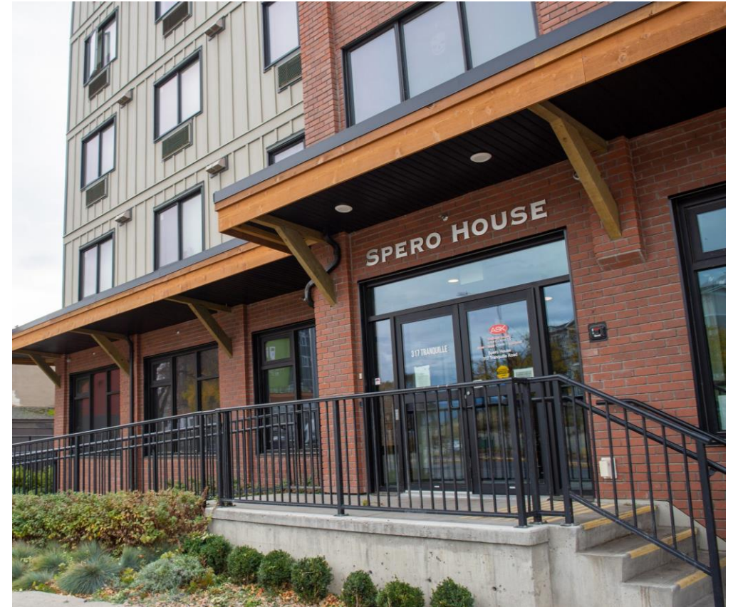
Spero House Supportive Housing, Kamloops
