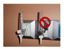
Thorpe tube Medical Air flowmeters and Oxygen flowmeters are visibly similar and have common outlet thread patterns which makes inadvertent errors in Air-Oxygen selection possible 1,2,3,5,6,7
